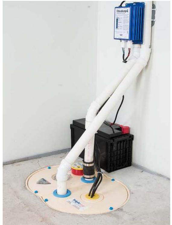
The pump should be tested and cleared of any debris on a regular basis. For additional protection, you can install a battery backup system with an alarm to ensure the pump functions properly in the event of a power outage. We recommend consulting with a certified plumber for options and installation.
